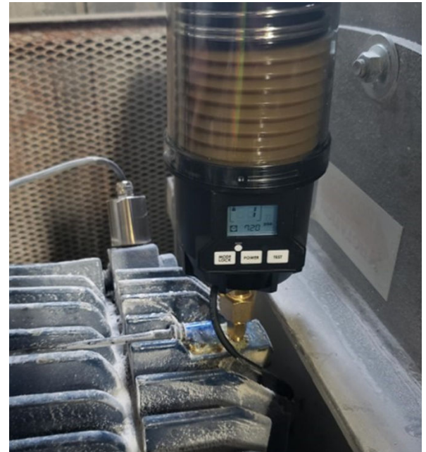
Figure 1 OnTrak system installed monitoring the real-time lubrication needs and health of the bearing on an air handler motor.
