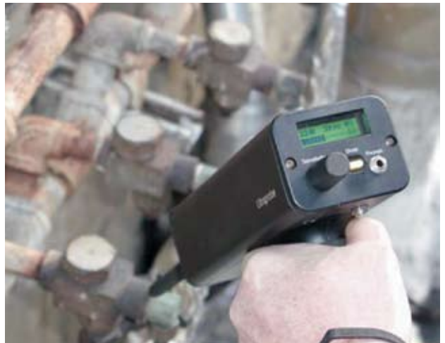
With energy costs increasing, ultrasound instruments can also be used to locate faulty steam traps and compressed air leaks.
